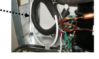
For <u>split level</u> "Bottle Filler ready" coolers, the tube to plumb in the Bottle Filler is packaged in the dummy unit or found inside the Bottle Filler.
