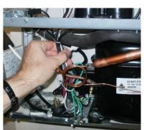
The tee and tube to the Bottle Filler are packaged with the Bottle Filler unit. One branch of the tee will supply the valve on the dummy unit, the other branch of the tee will connect to the Bottle Filler.
